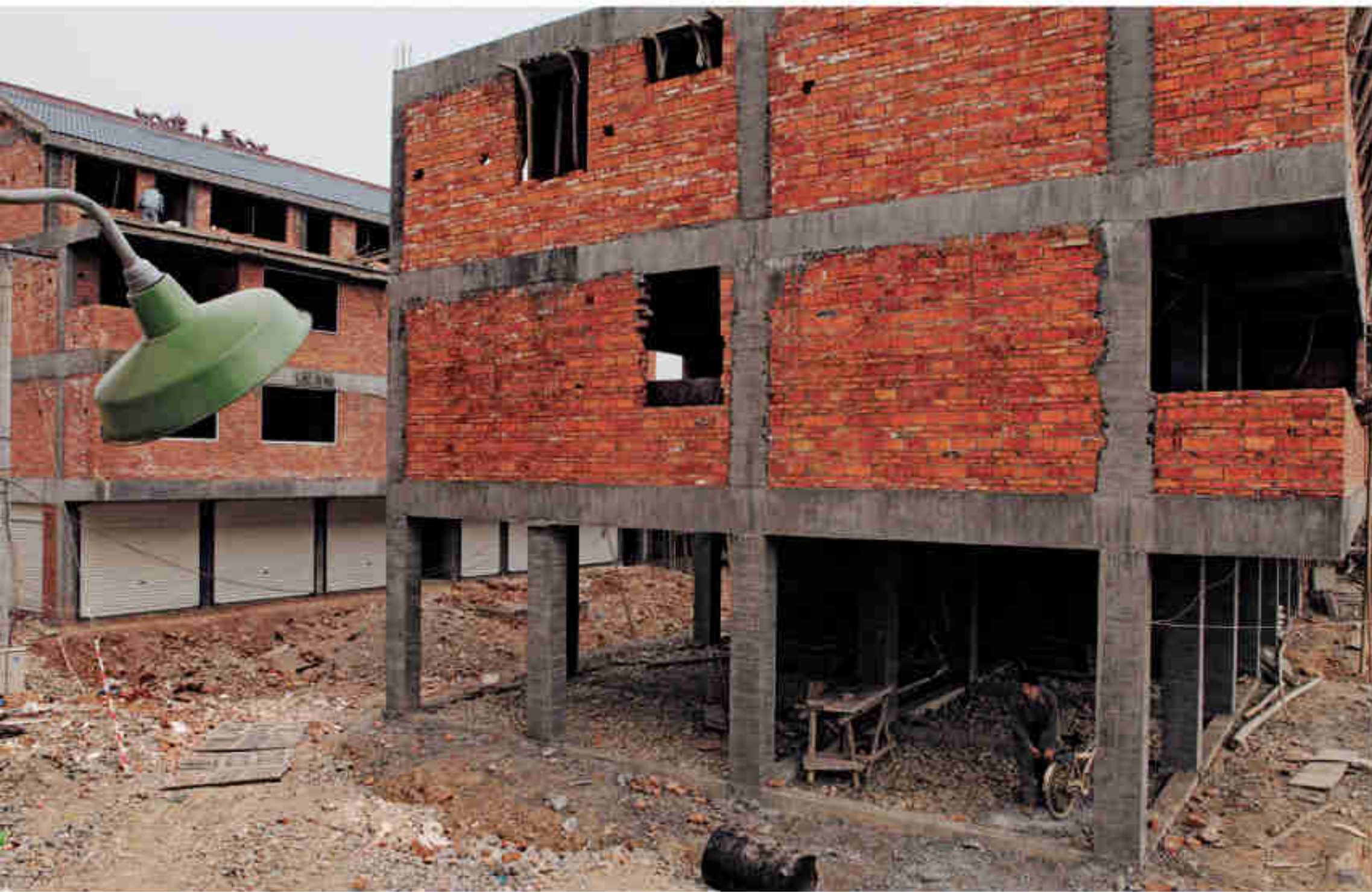
FEBRUARY 2006: SHELL FINISHED
